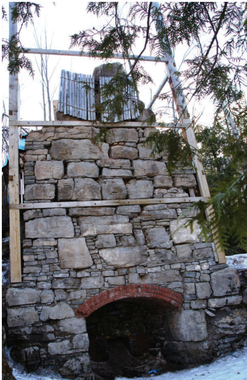
▲ The front face of the Draw Kiln after restoration and stabilization to date. The Society would like to restore the structure to the top wooden rail. PHOTO BY MIKE DAVIS.
