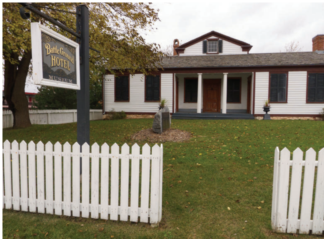
▲ Fralick's Tavern, constructed in 1836 on the site of the Battle of Lundy's Lane, is now a museum.
